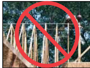
Truss spacers are insufficient as Lateral Restraint and Bracing.
