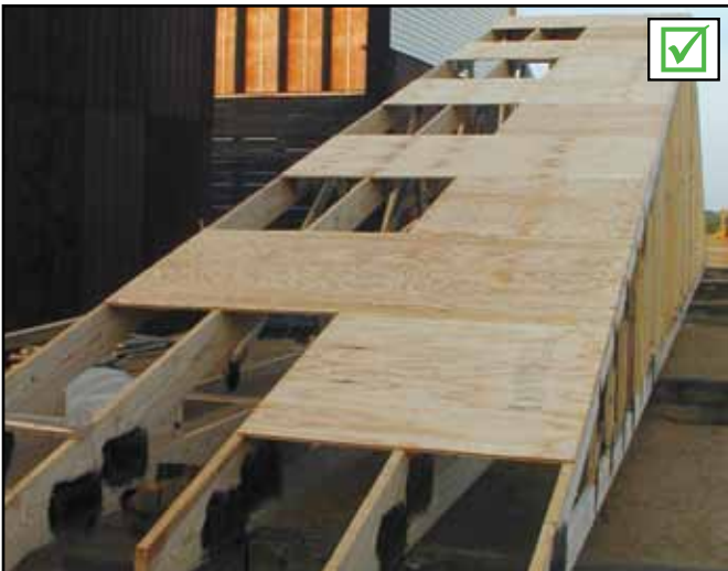
Install Structural Sheathing as soon as the first "set" of Trusses have been properly plumbed, restrained and braced. Begin at the heel and alternate 4'x8' and 4'x4' sheets up to the peak.
